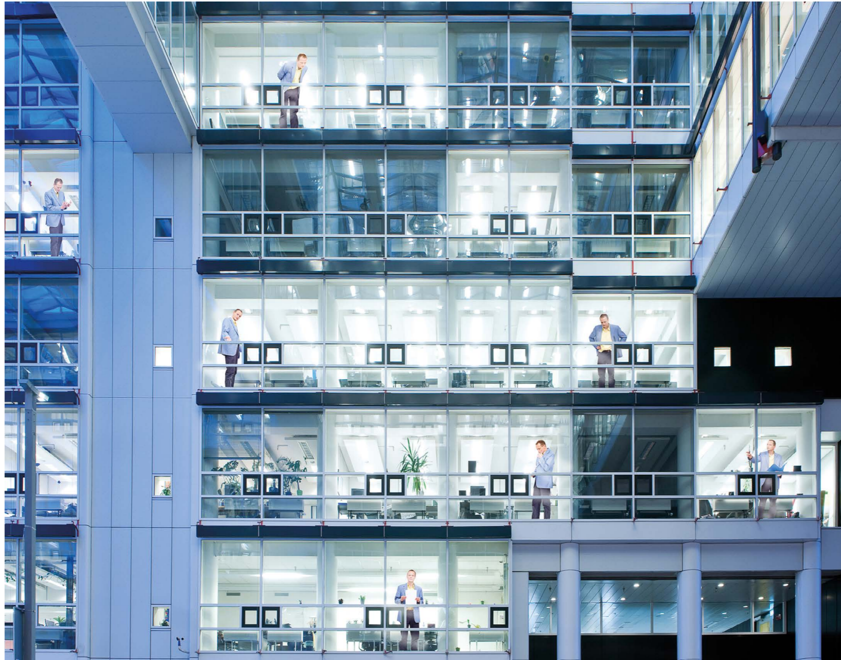
The presence detector switches on the luminaires in the selected spaces when somebody occurs there and thus when the illumination is really necessary.
